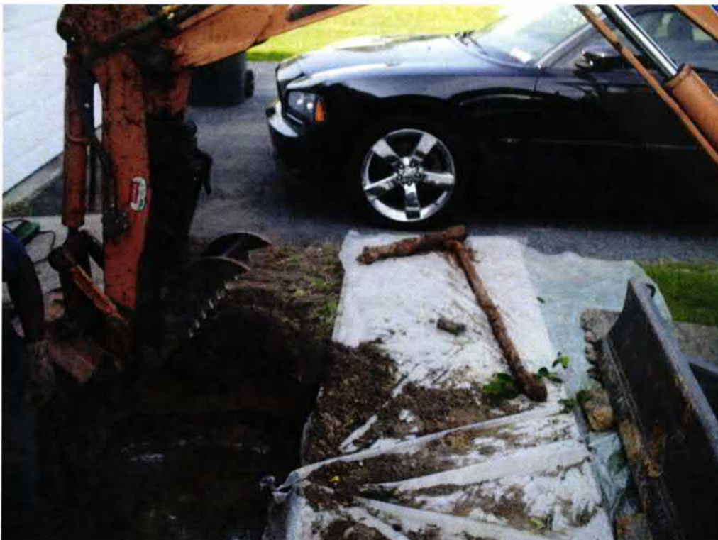
Picture 2: UST 311Ash removal in progress.
